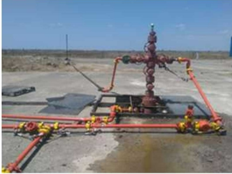
Fig 7. Wellhead set-up circulating, cementing, flaring
