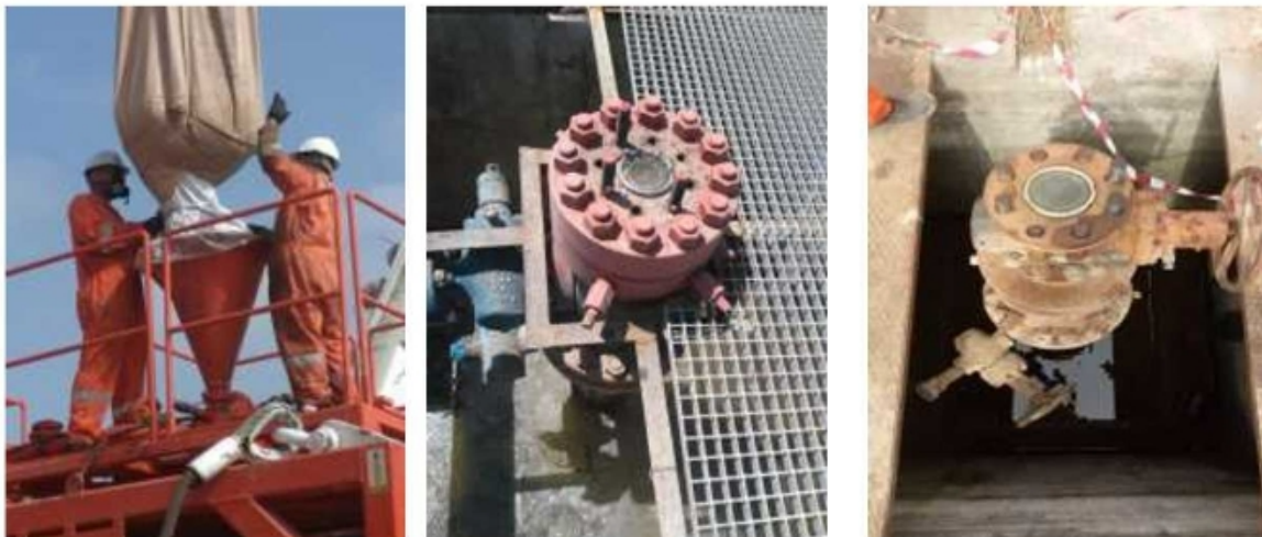
Fig 13, 14, 15 : Fully cemented tubing side as a result of hard work by the cementing team
