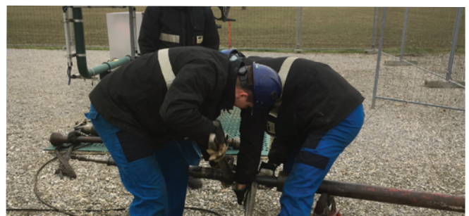
PulseEight ICV installation
