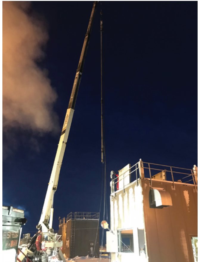
Rig up and installation of PulseEight ISV
