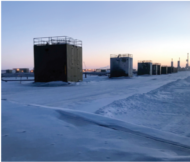
Prudhoe Bay pad wellhouses
